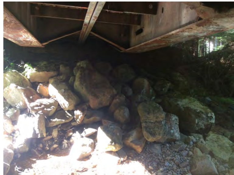
Left Bank Abutment when facing downstream
