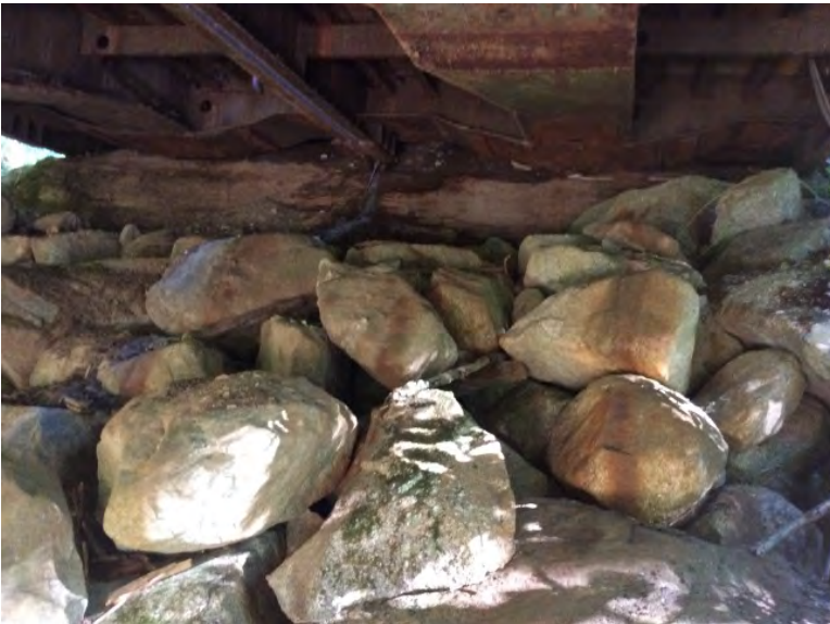
Right Bank Abutment when facing downstream
